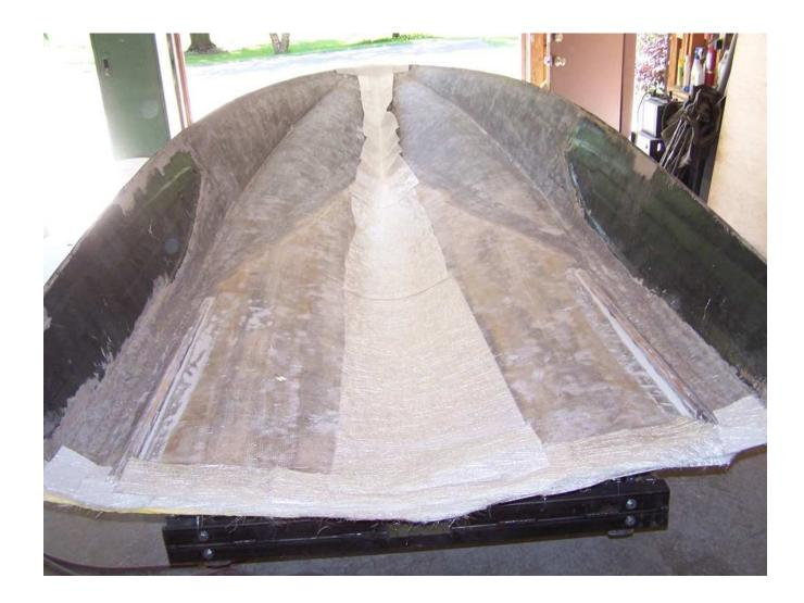
One layer over the entire hull, and extra material along the keel and transom pad. (Different hull than previous pictures.)
