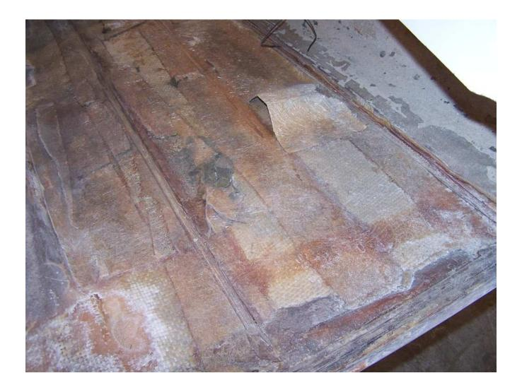
Grind smooth and remove any loose laminates. (dirty job... wear gloves, respirator and coveralls!)
